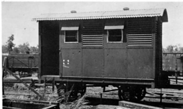
Shrapnel holes can be seen clearly in the sides of the leper van. The van saw little use during the war as most of its customers 'went bush' after the first air raids. (Photo: Elmore Schultz)
